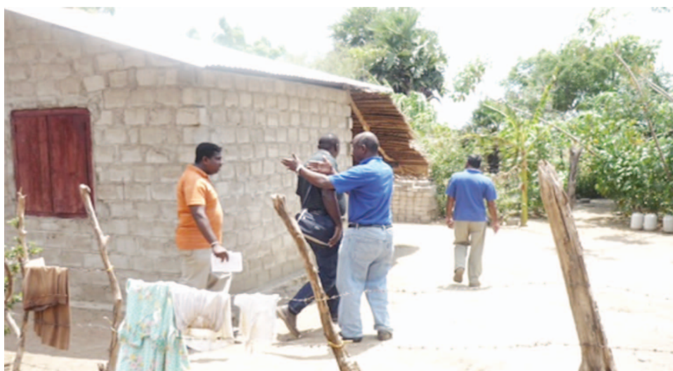
“OfERR-UNHCR repair of damaged homes - Muthur, Trincomalee”
